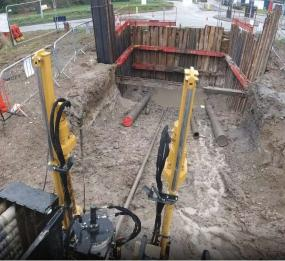
The client discussed scenarios and capabilities with CMS in liaison with specialist engineers and designers to find resolution. It was agreed to increase drill depths until the obstructions were cleared, when cleared, the drill depth was to be further increased to ensure the pipes were installed clear of the obstruction.
